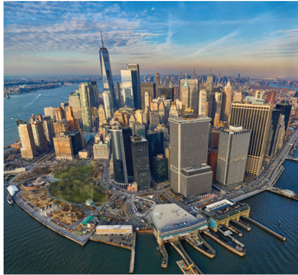
9.2.6 Oblique aerial photograph of New York City's Financial District, located on the southern end of Manhattan
