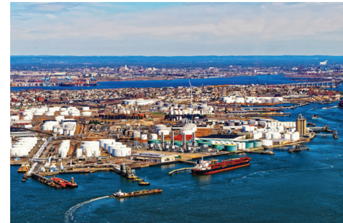
9.7.2 New York-New Jersey container terminals and Newark Liberty International Airport
