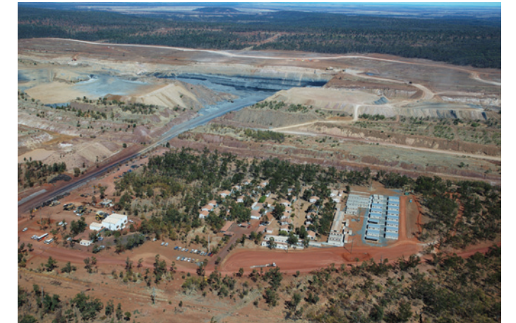
6.1.20 Remote mining camp, Central Queensland
