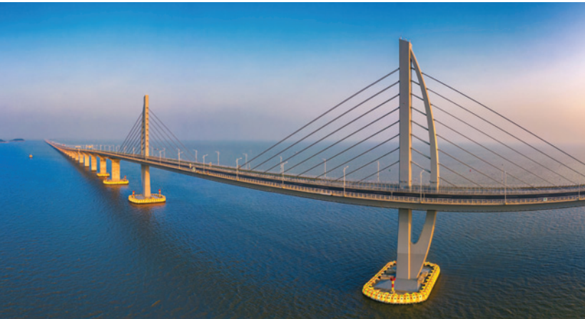
6.1.6 The Hong Kong–Zhuhai–Macau Bridge in China is a 55-kilometre bridge–tunnel system consisting of a series of three cable-stayed bridges, an undersea tunnel, and four artificial islands. It is the longest such crossing in the world.
