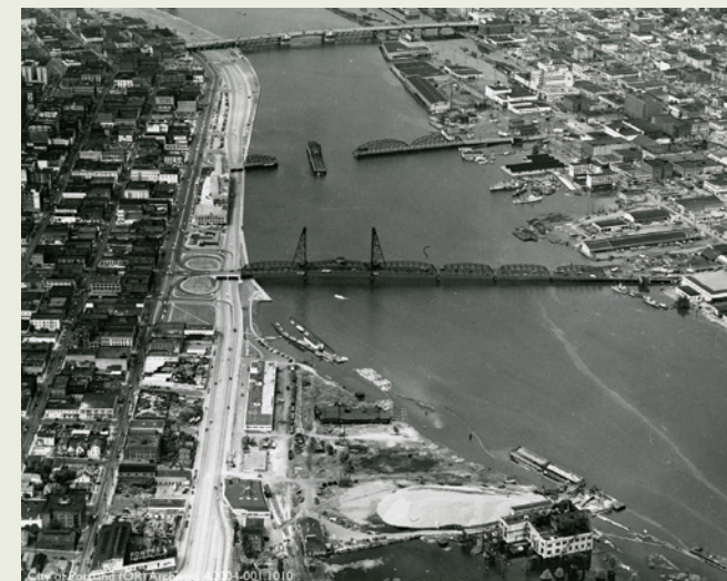
6.5.6 Portland's Harbor Drive under construction
