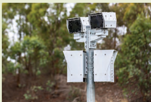
FIGURE 3.1.6 Speed cameras on poles.
