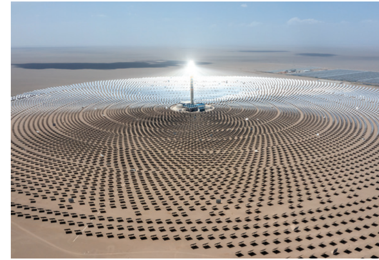
5.1.9 This solar thermal power station is in north-west China. The total reflection area of the power station's mirror field is 1.4 million km 2 . When the sun shines down, the heliostat will reflect and concentrate the light on the top of the heat absorption tower.
