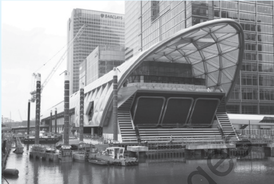
FIGURE 1.3 A Crossrail station being built in central London
