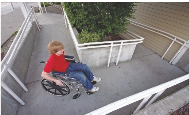
This shows an excellent example of an access route for a wheelchair. Notice the easy slope and dual-level railing?
