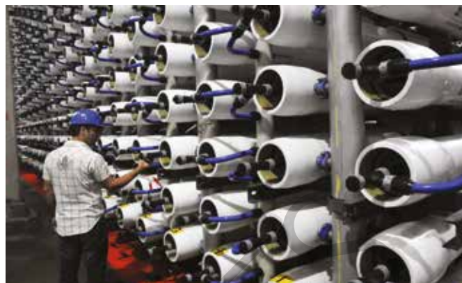
FIGURE 4.4.5 Reverse osmosis desalination plants have been built near Perth, Sydney, Melbourne and the Gold Coast to treat seawater and make it into drinking water.
